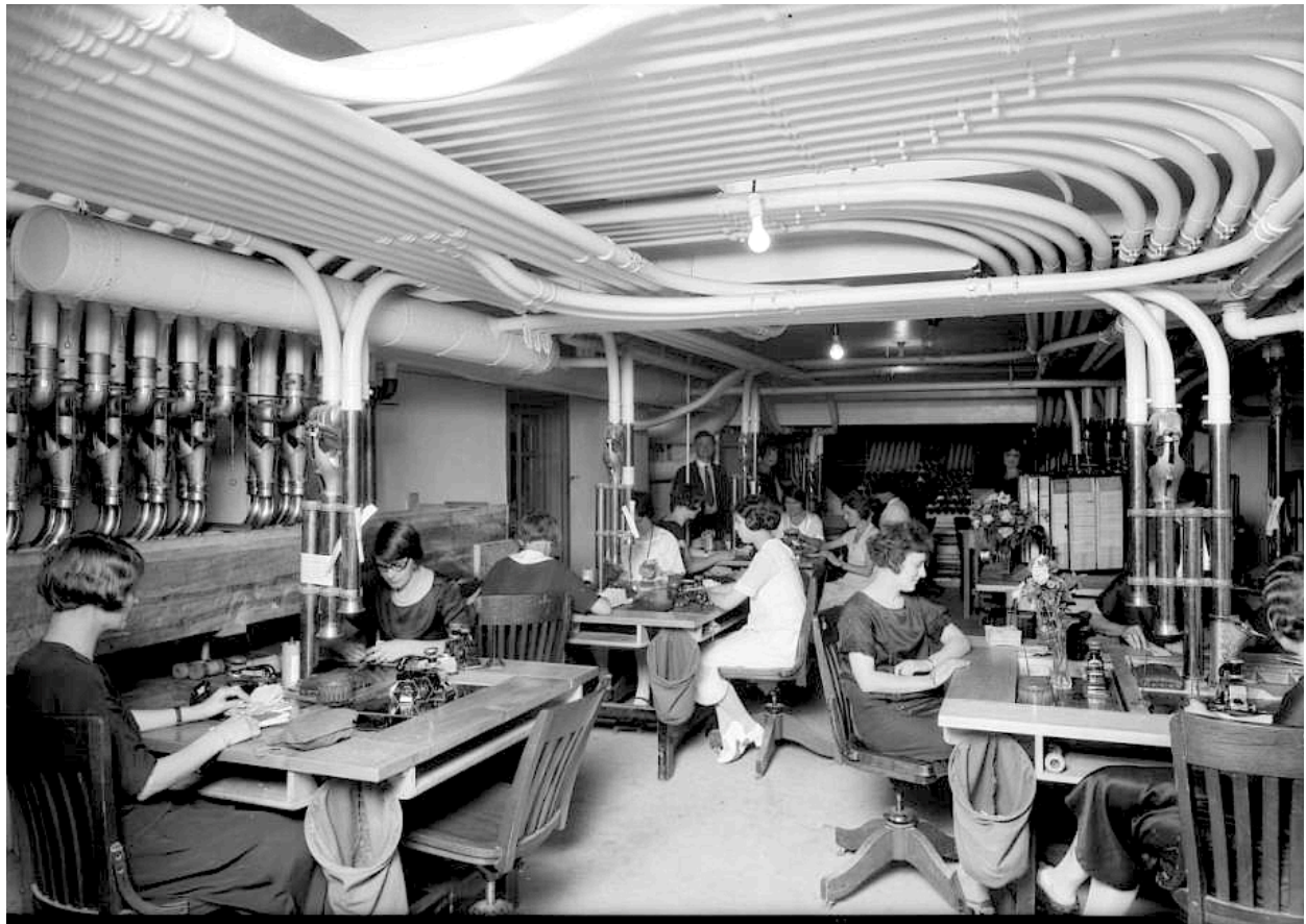
Figure 5.1 – Pneumatic tube system for a department store on Broadway in New York City (1925)
